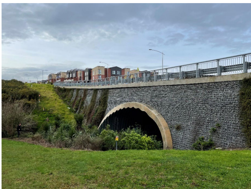
Figure 5: Culvert under Murphys Park Drive.
